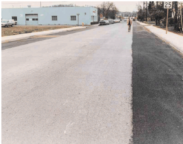
Above: An RCC pavement. This material has very much more cement than RCC for Dams.
