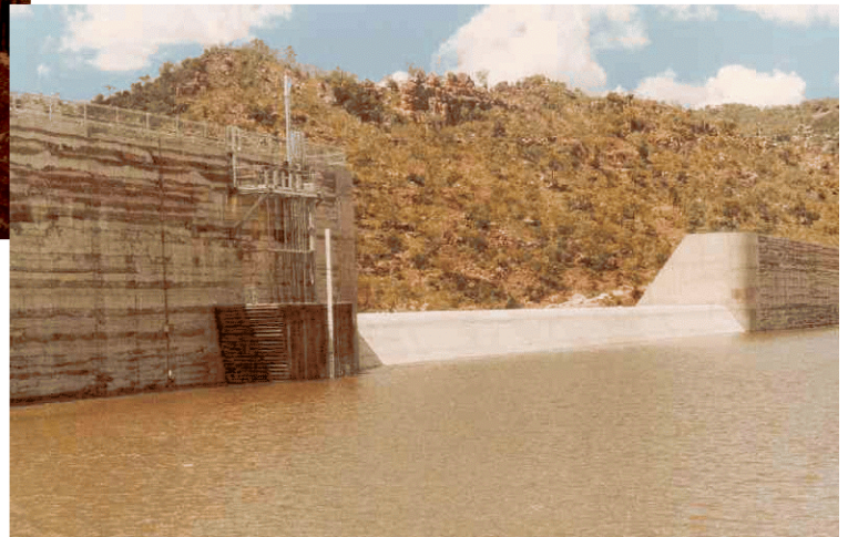
An early low paste RCC dam, Copperfield Northern Queensland, Australia. The upstream face was conventional concrete placed against forms. The downstream face of the dam was unformed except for the spillway which was conventional concrete. This 40 metre high dam contained 140,000 cubic metres of RCC and 16,000 cubic metres of conventional concrete. It was built in 1984 over a period of 16 weeks. The RCC was mixed with excellent uniformity by two ARAN ASR200 continuous mixing plants.
