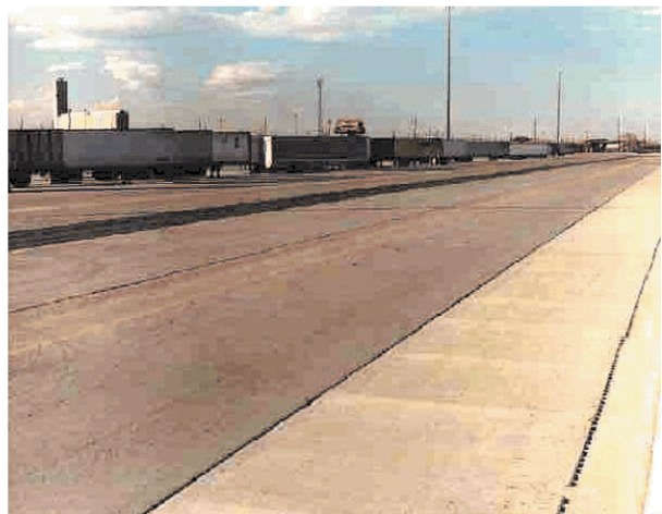
Above: An RCC pavement used for large freight transfer terminal USA.
