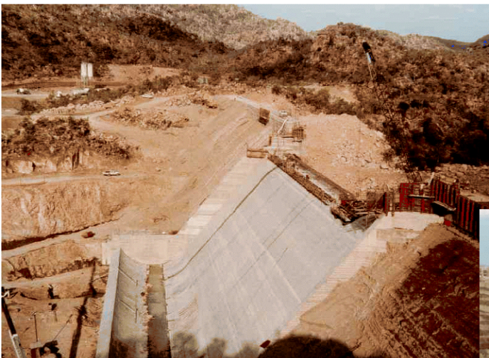
An early low paste RCC dam, Copperfield Northern Queensland, Australia. The upstream face was conventional concrete placed against forms. The downstream face of the dam was unformed except for the spillway which was conventional concrete. This 40 metre high dam contained 140,000 cubic metres of RCC and 16,000 cubic metres of conventional concrete. It was built in 1984 over a period of 16 weeks. The RCC was mixed with excellent uniformity by two ARAN ASR200 continuous mixing plants.
